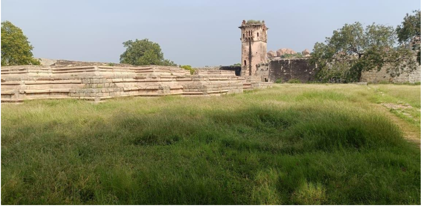
Before cleaning the vegetation at the premises of the Zanana Encloser at Kamalapura
