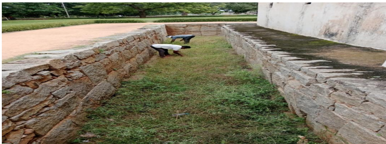
During cleaning of the vegetation at the Queens Bath at Kamalapura
