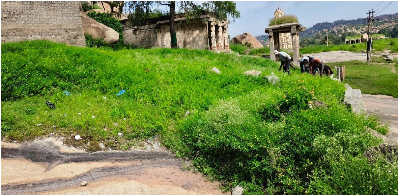
Before cleaning the vegetation at the Kadalekalu Ganesha Temple at Hampi
