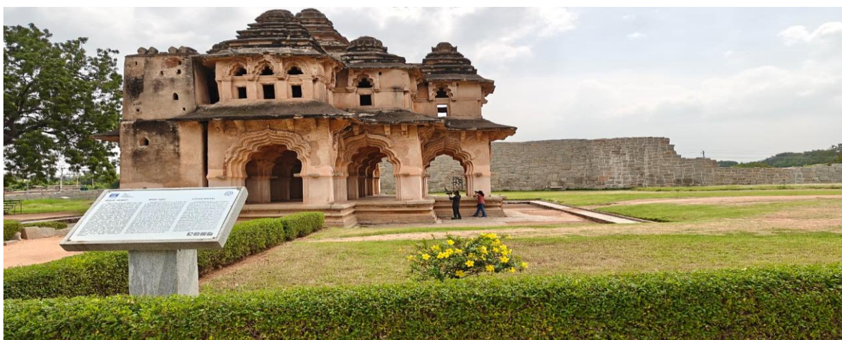
After cleaning the vegetation at the premises of the Zanana Encloser at Kamalapura
