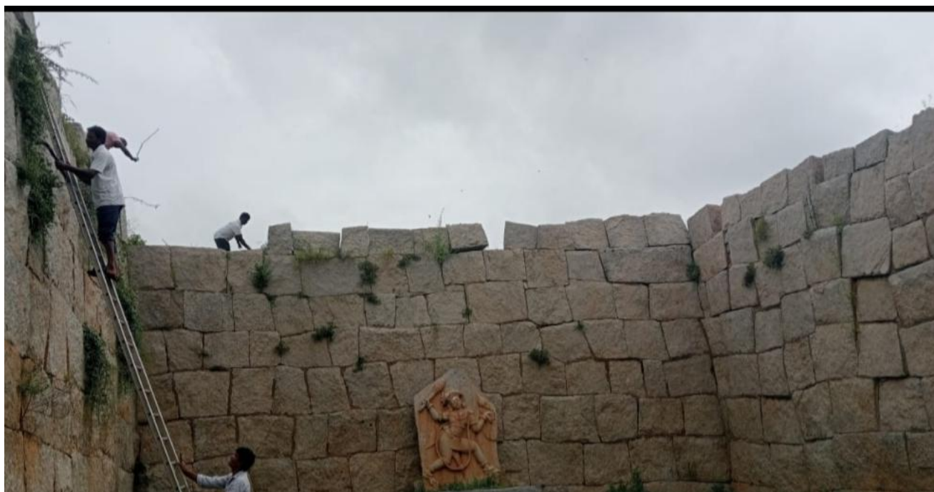
During cleaning of the vegetation on the walls of the Bhima's gateway at Kamalapura
