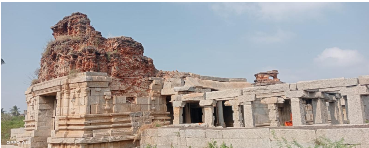
After cleaning the vegetation at the Vishnu Temple at Kamalapura
