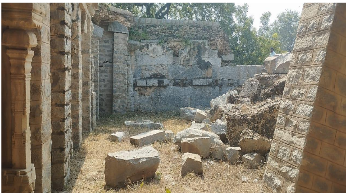
After cleaning the vegetation at Achutadevaraya Temple at Venkatapura
