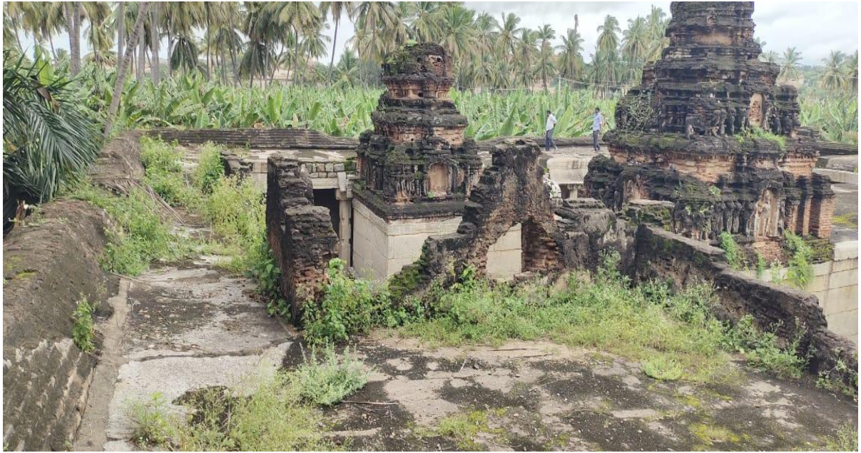
Before cleaning the vegetation at the Chandikeshwara Temple at Krishnapura
