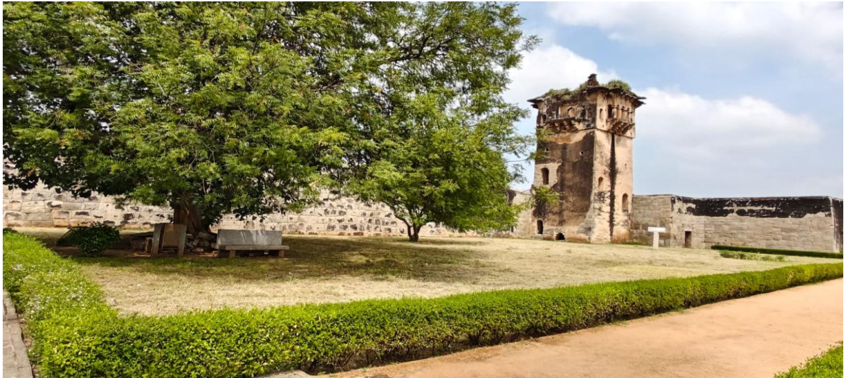
After cleaning the vegetation on the premises of the Zanana Encloser near the Southeast watch Tower at Kamalapura
