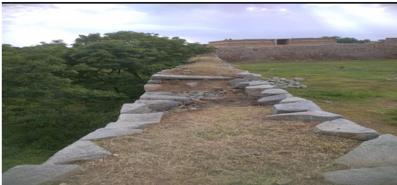
After cleaning the vegetation in the Royal Enclosure area at Kamalapura
