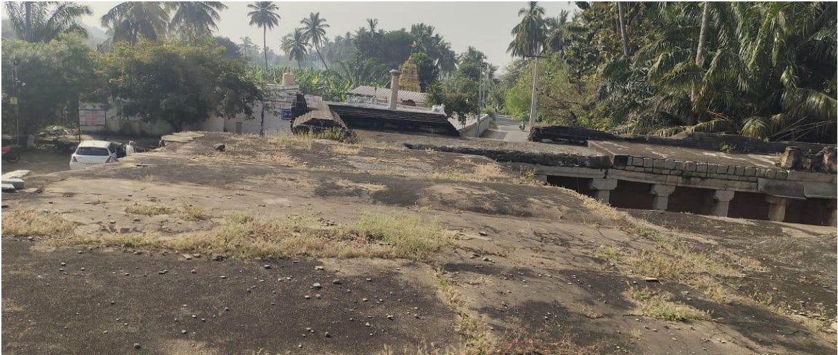
Before cleaning the vegetation at Chandikeshwara Temple at Krishnapura
