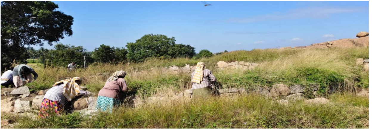
During cleaning of the vegetation at the Sasivekalu Ganesha Temple at Krishnapura
