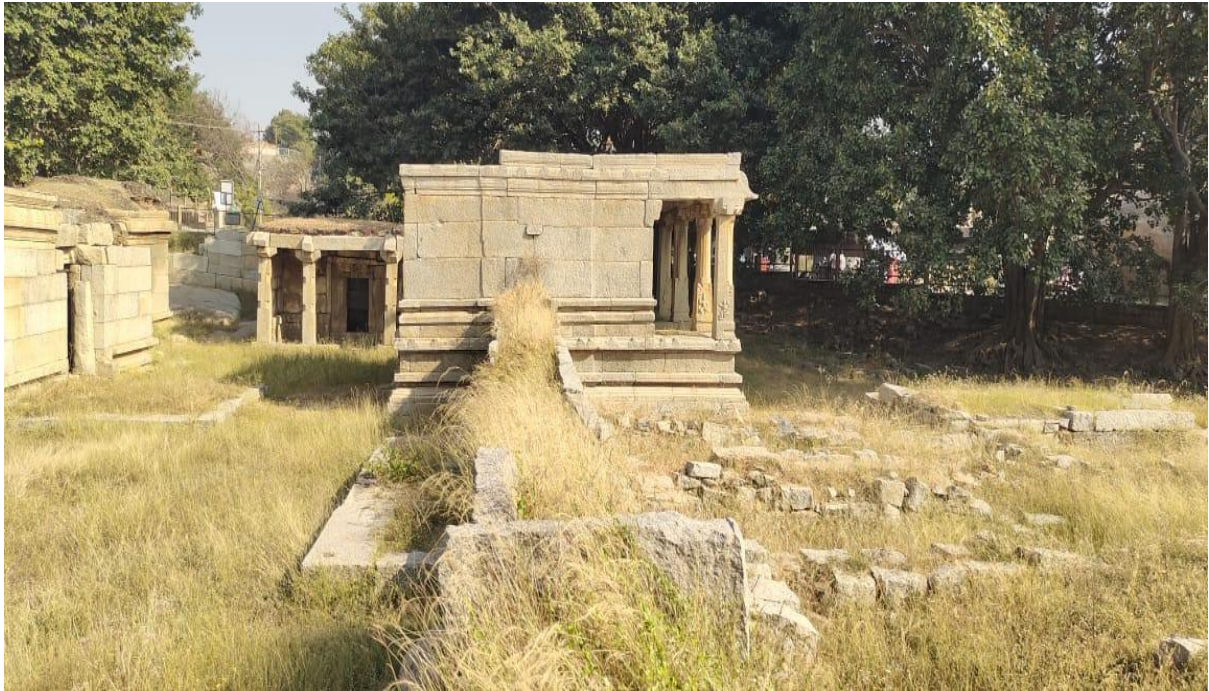
Before cleaning the vegetation at Prasanna Narasimha Temple at Krishnapura
