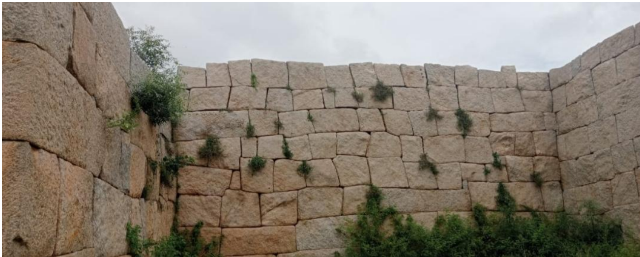
Before cleaning the vegetation on the walls of the Bhima's gateway at Kamalapura
