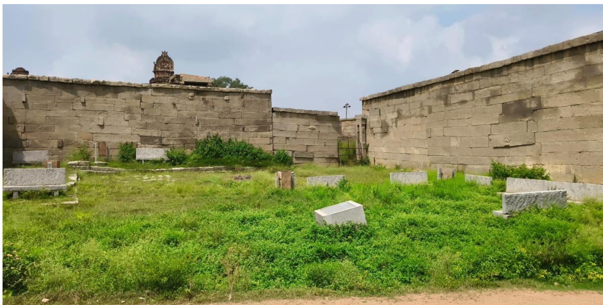
Before cleaning the vegetation at the Krishna Temple at Krishnapura
