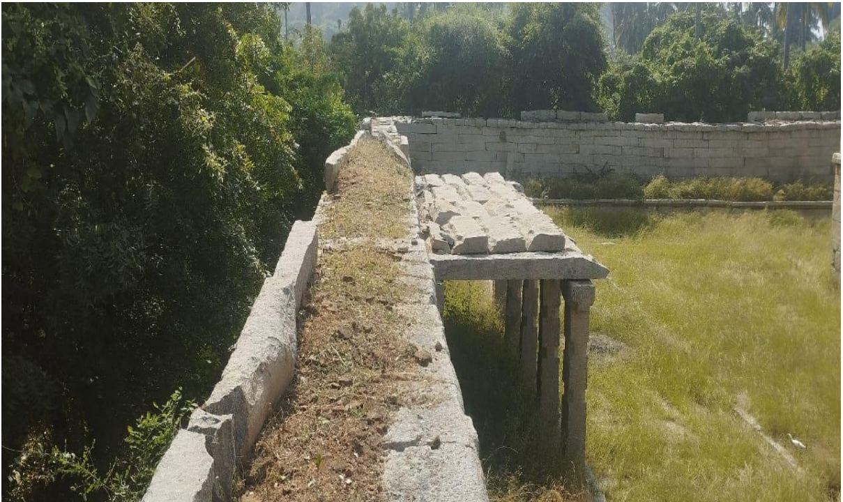
After cleaning the vegetation at Achutadevaraya Temple at Venkatapura
