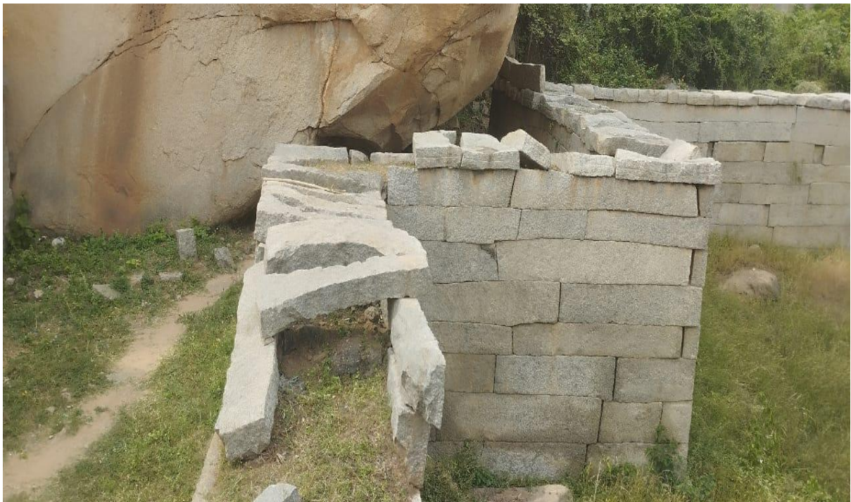
After cleaning the vegetation at Achutadevaraya Temple at Venkatapura
