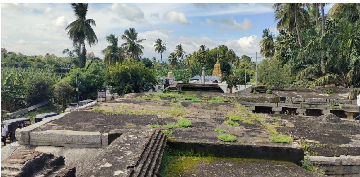
Before cleaning the vegetation at the Chandikeshwara Temple at Krishnapura
