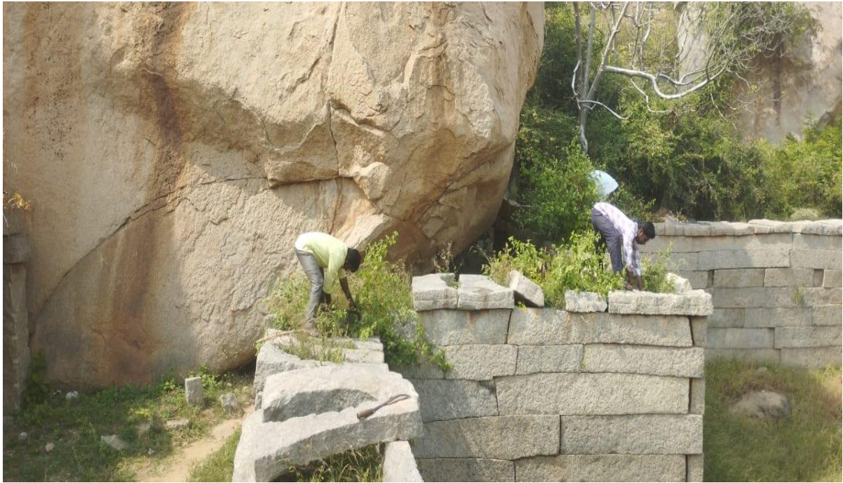
During cleaning of the vegetation at Achutadevaraya Temple at Venkatapura
