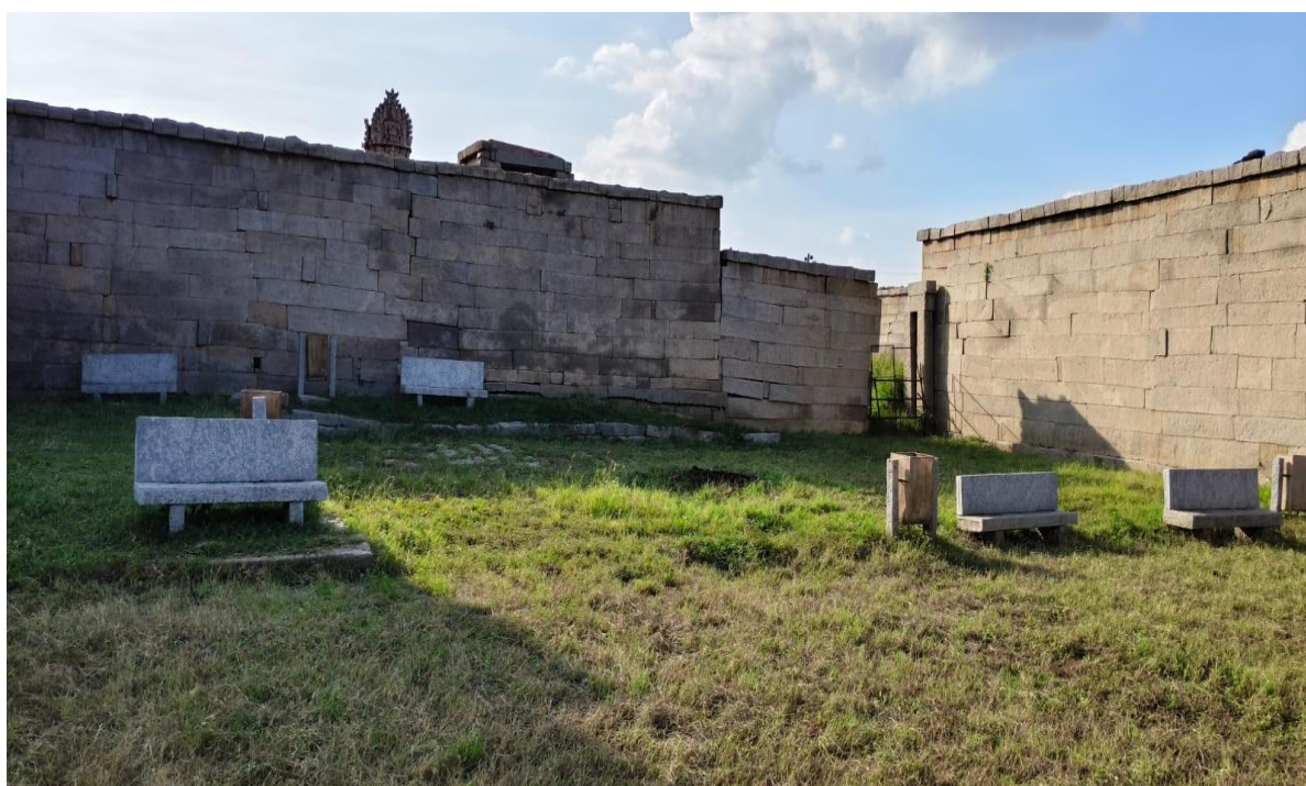
After cleaning the vegetation at the Krishna Temple at Krishnapura
