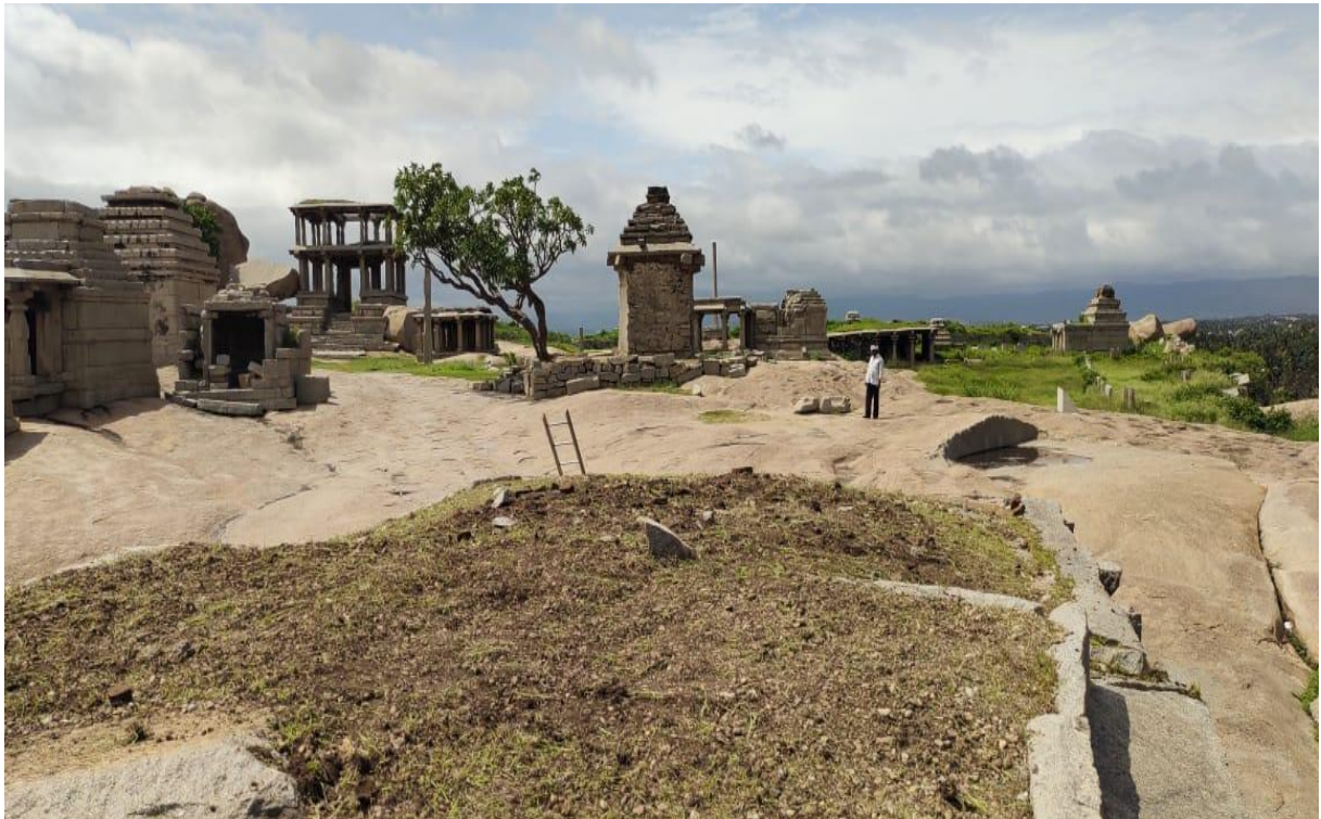
After the cleaning of the vegetation at the premises of the double-storied Mantapa at Hampi
