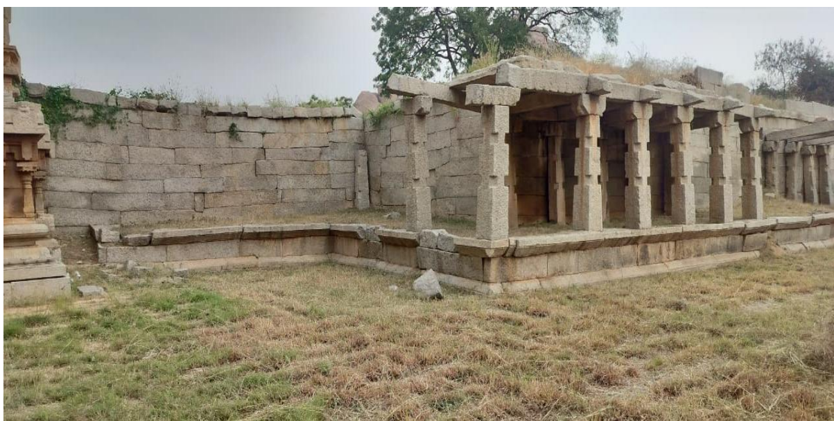
After cleaning the vegetation at Achutadevaraya Temple at Venkatapura
