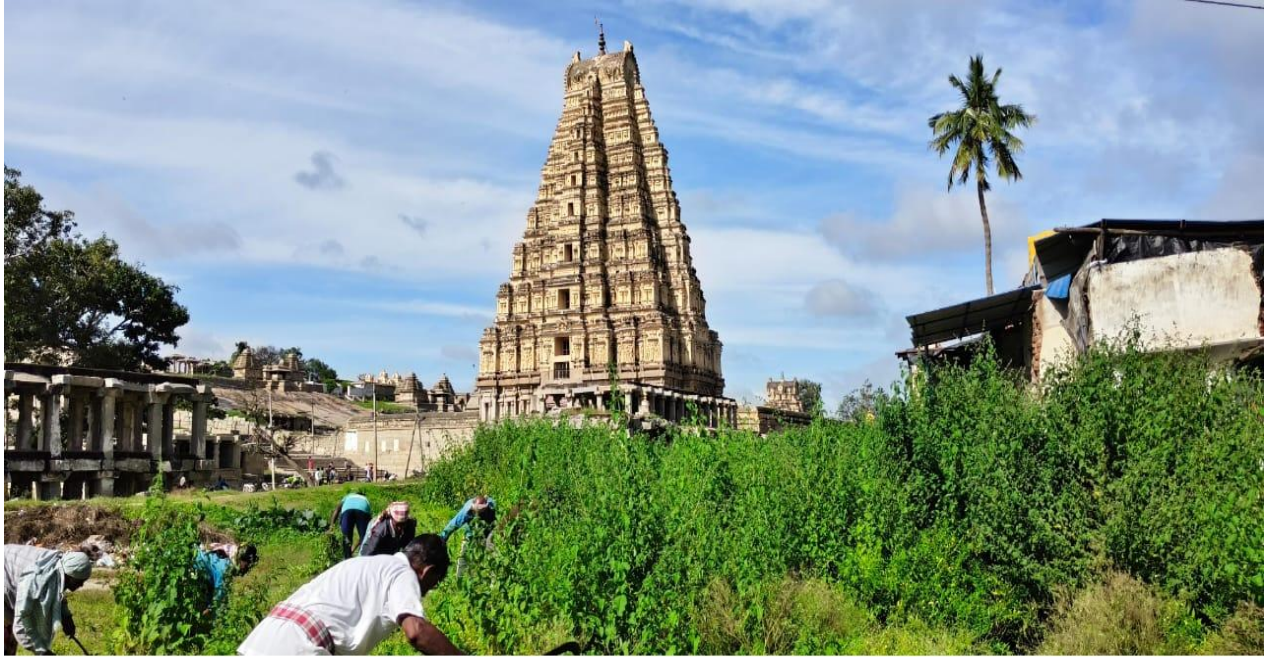
Before cleaning the vegetation at the Bazar area of the Virupaksha Temple at Hampi
