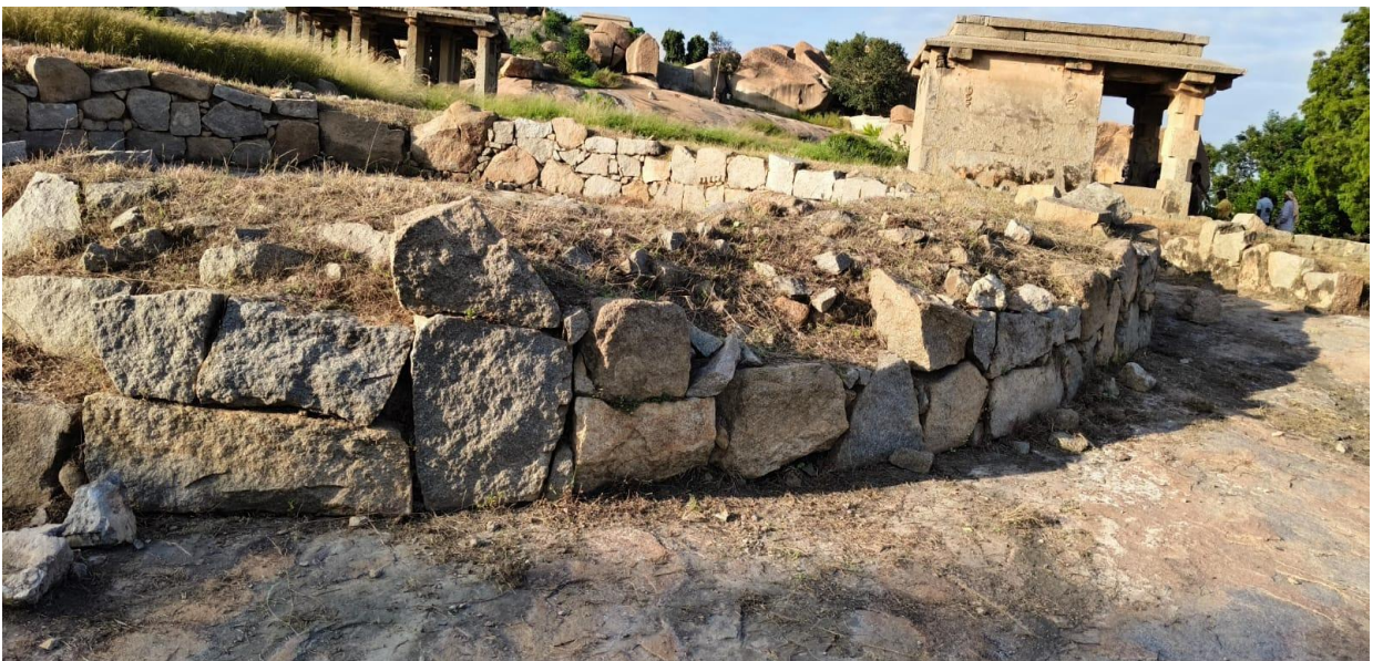
After cleaning the vegetation at the Sasivekalu Ganesha Temple at Krishnapura
