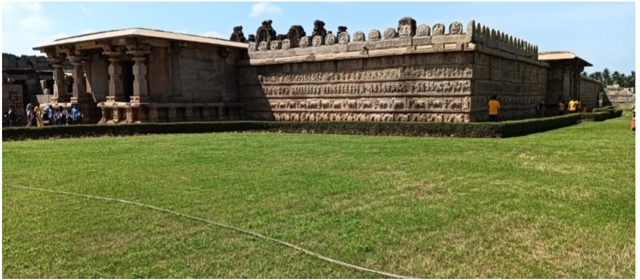
After cleaning the vegetation at Hazararama temple at Kamalapura
