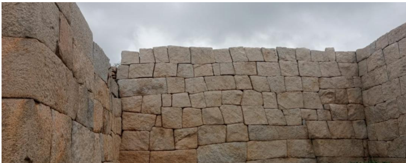
After cleaning the vegetation on the walls of the Bhima's gateway at Kamalapura
